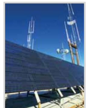
PV used for a remote telecommunication station
