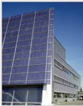
PV system integrated in a facade
