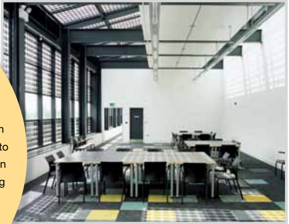
PV cells used as sunshade in an office building, UK
