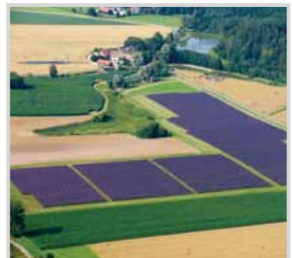
Large photovoltaic power plant in Bavaria
